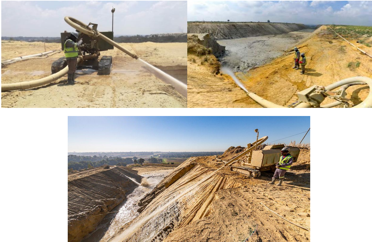
Figure 2-1: Mobile Tracked Hydraulic Monitor on a Tailings Facility in South Africa (Kongiwe, 2025).
