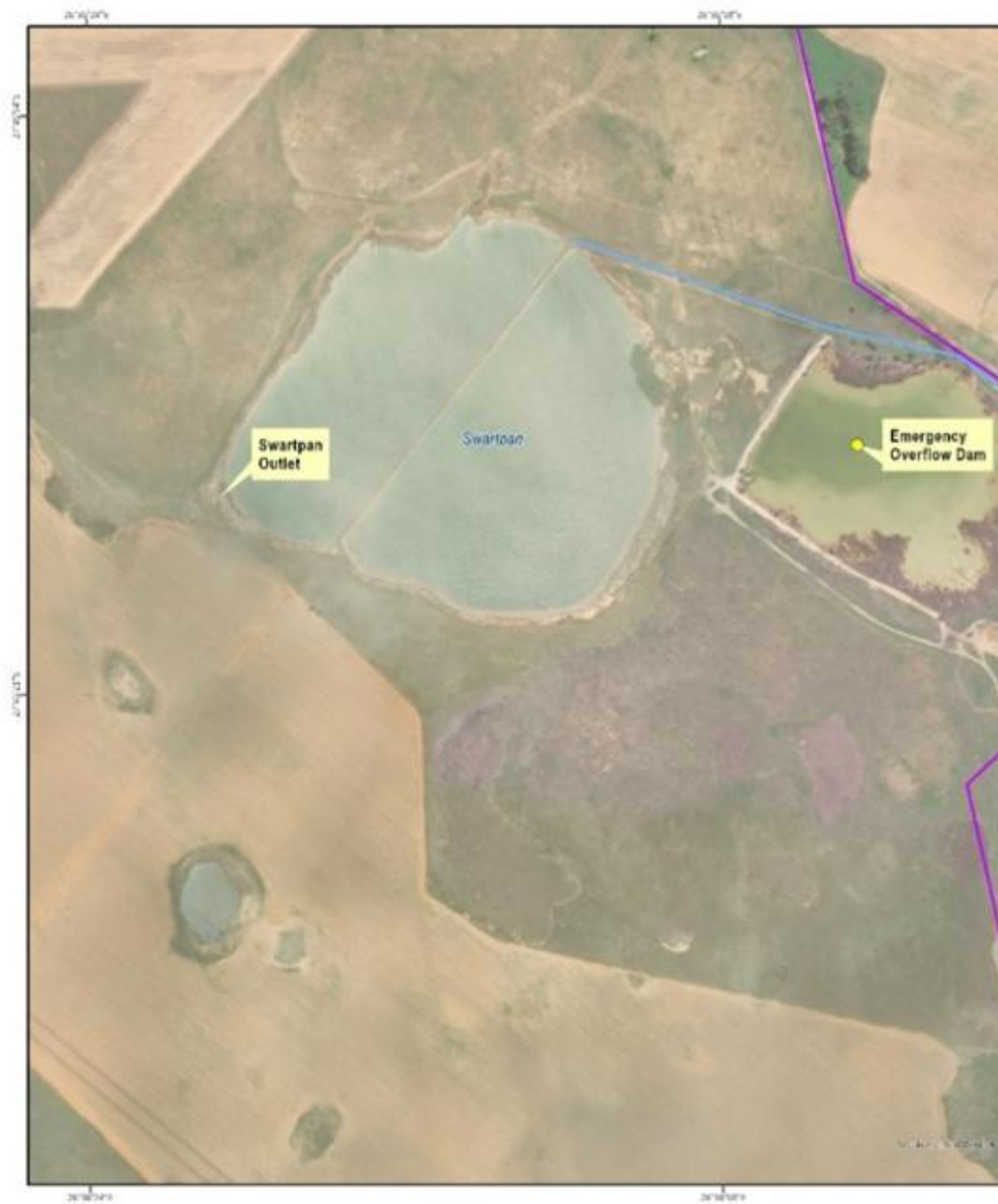
Figure 5-4). The purpose of the channel is assumed to be to bypass the “clean” stormwater runoff around the “dirty” mine infrastructure. This open channel is currently completely overgrown (See Figure 5-5).
