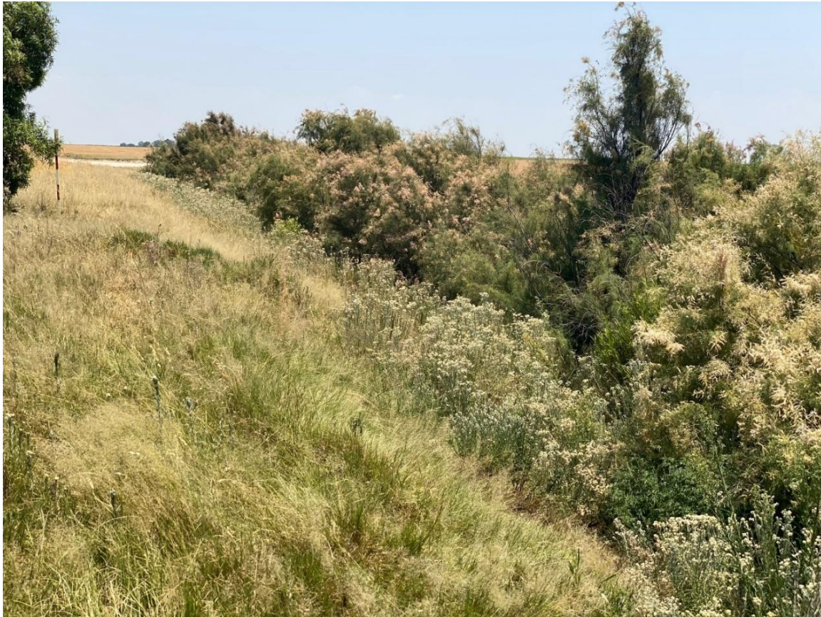
Figure 5-5: Open Trench to Swartpan, Completely Overgrown
