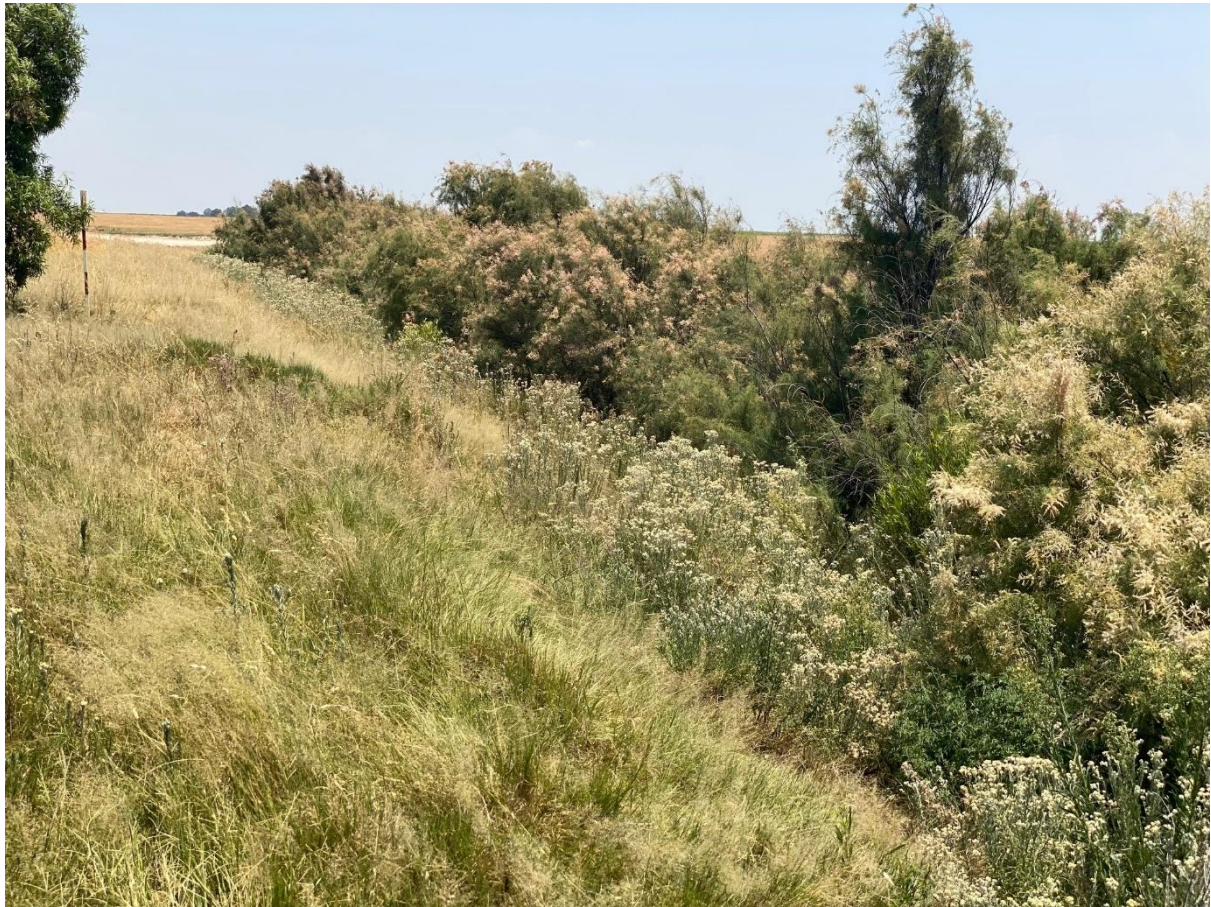
Figure 17: Open Trench to Swartpan, completely overgrown
