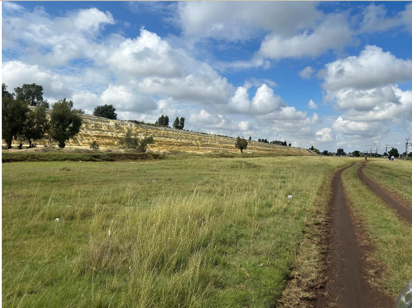
Access road leading to the 6L14 TSF on the western side: 26°12'58.04"S 28°28'10.03"E
