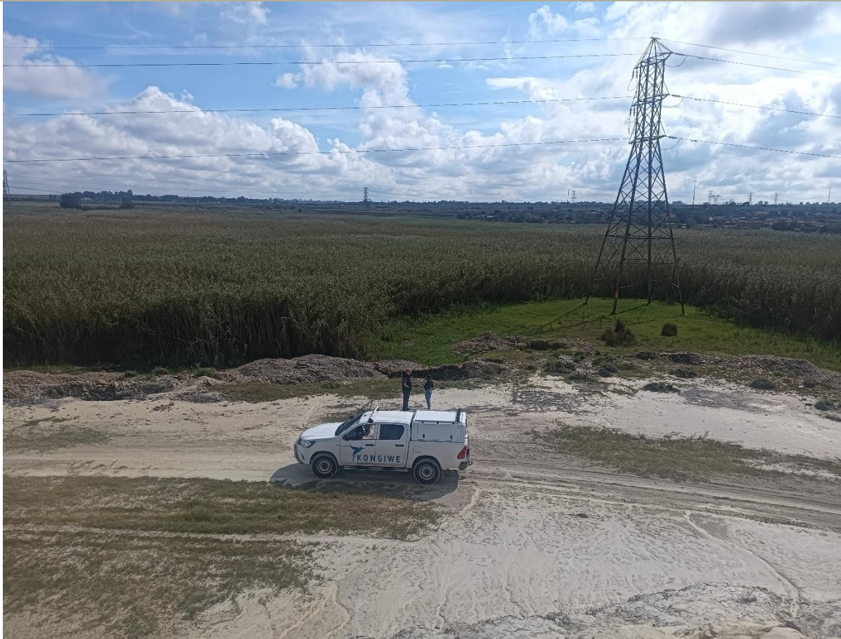
View of the existing powerline and watercourse located on the northern side of the TSF: 26°12'31.61"S 28°28'42.71"E
