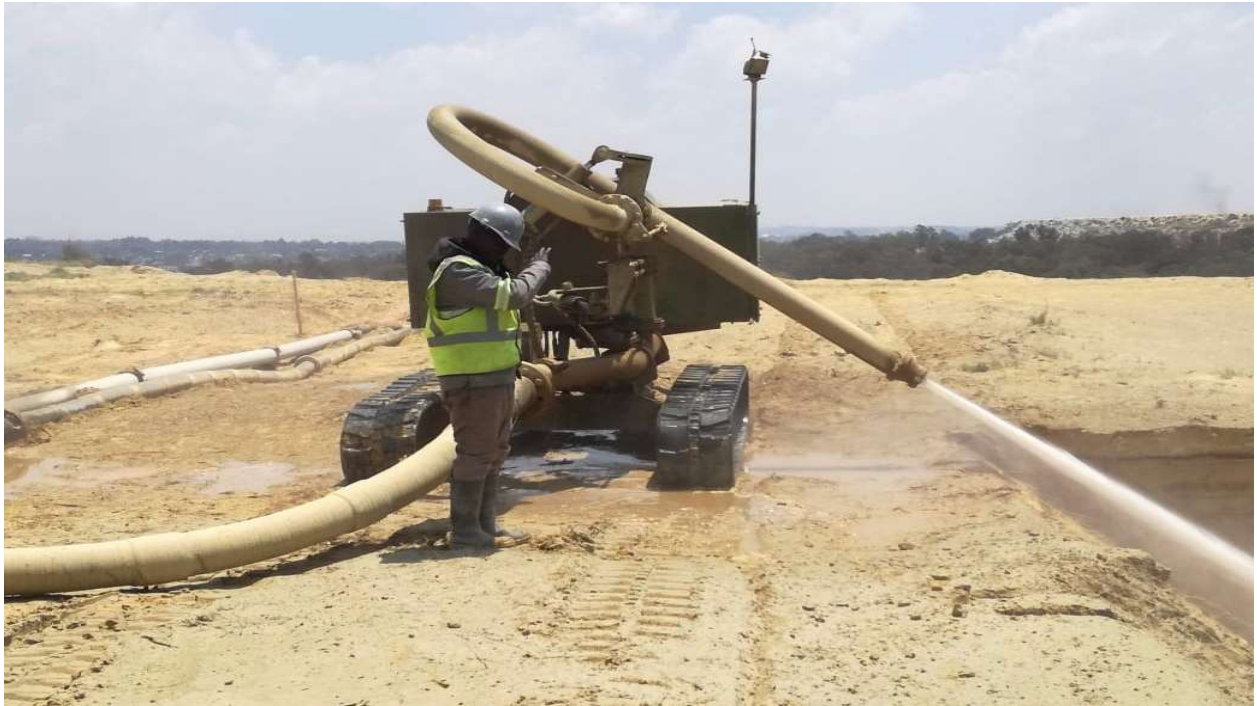
Figure 2-5: Mobile tracked hydraulic monitor on a tailings facility in South Africa
