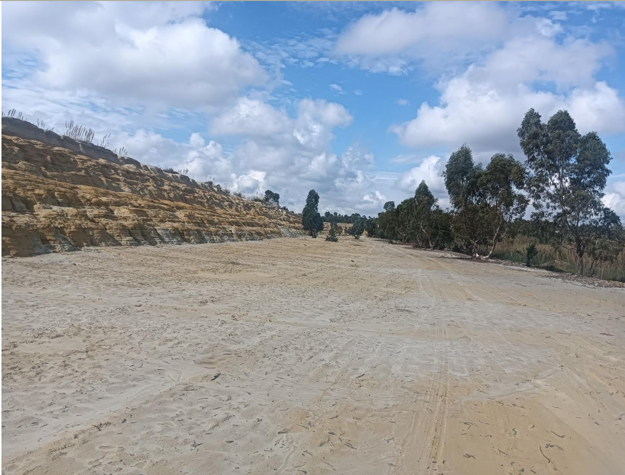
Cleared and sandy area beside TSF slope: 26°12'31.62"S 28°28'36.14"E
