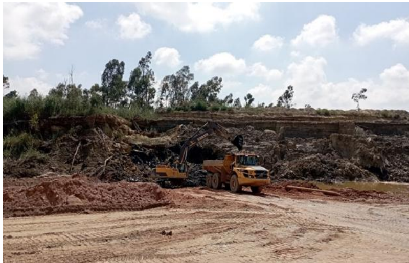
Figure 4: Example of a Truck and Shovel Reclamation
