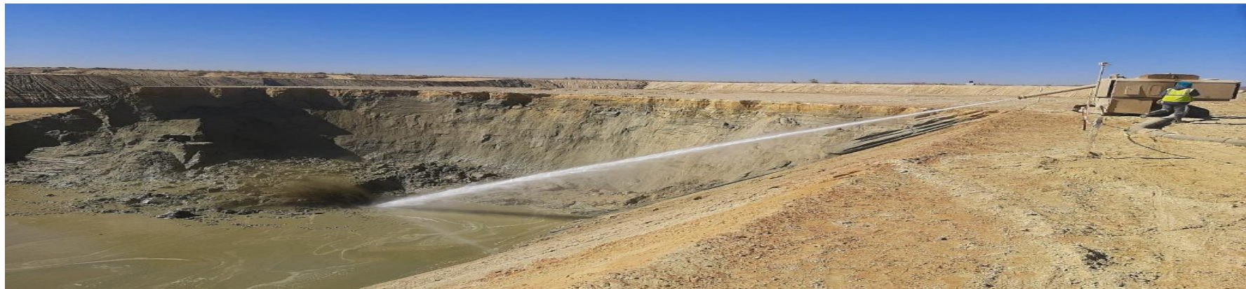
Figure 5: Example of Hydraulic Reclamation
