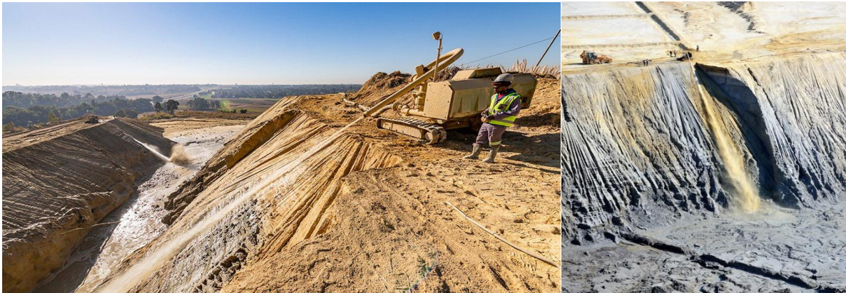
Figure 3: Mobile tracked hydraulic monitor on a tailing's facility in South Africa
