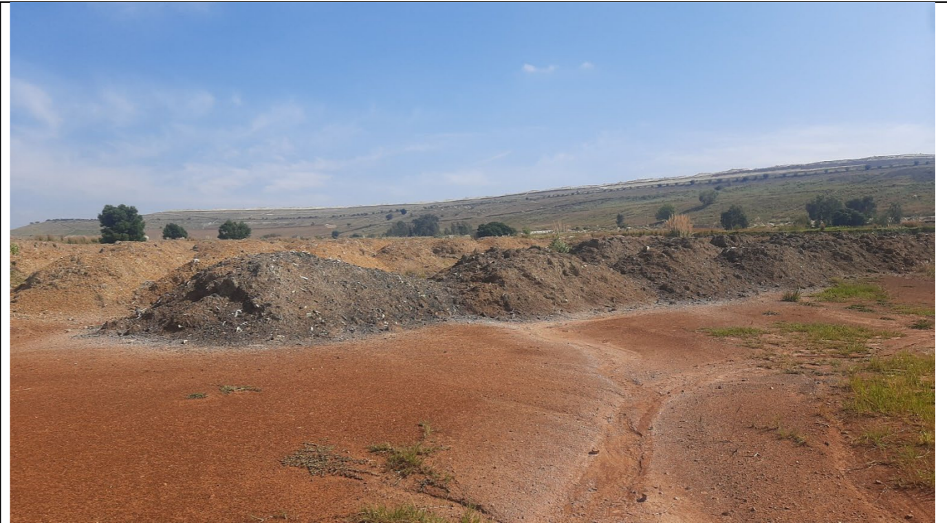
Cladding stockpiles for the Brakpan TSF
