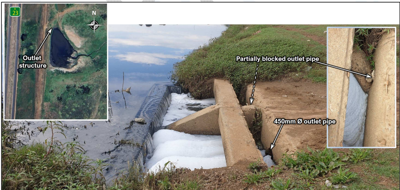
FIGURE 5: ATTENUATION DAM OUTLET STRUCTURE
